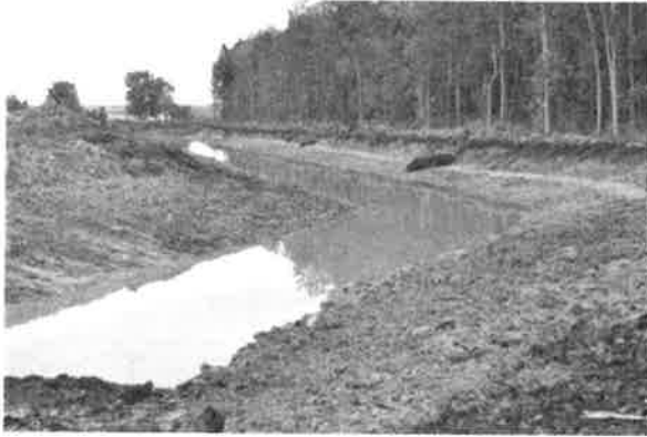
Figure B11-4. A dewatered channel with a littoral shelf on the right side of the channel.
