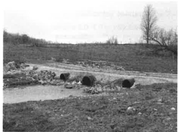
Figure B3–7. A low level crossing.
