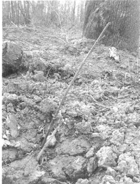
Figure B11-10. A live cutting placed in the stream bank.
