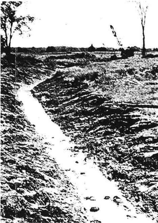
Open drain under construction.
