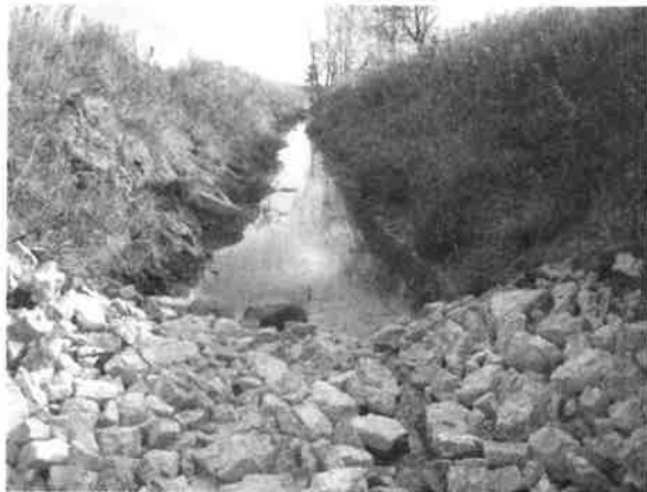
Figure B7-7. A rock check dam installed in a drain.
