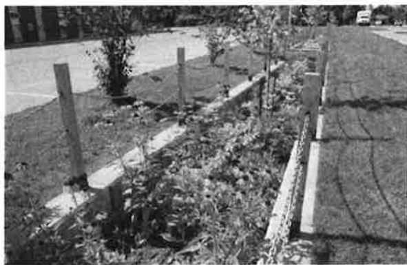
Figure B5-1. A bioswale is an example of a LID technique used to reduce surface water runoff.
