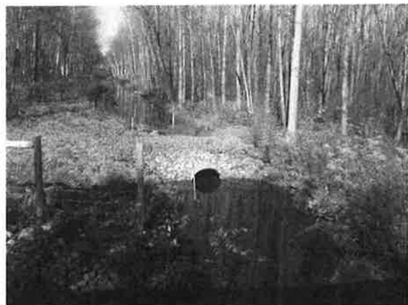
Figure B8–2. A wetland drain restoration project.
