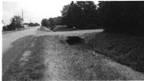
Figure B10–1. An open-bottom crossing/pipe arch.
