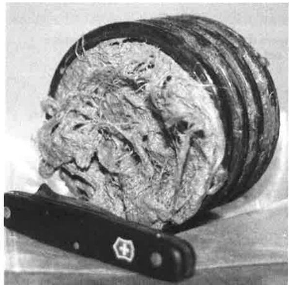
Figure B9-5. A tile plugged with tree roots.
