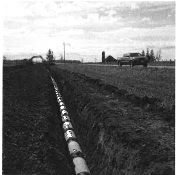
Figure B10–11. Installation of a rural pipe drain.
