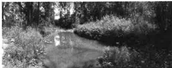
Figure B11-9. Live crib wall 2 years after construction.
