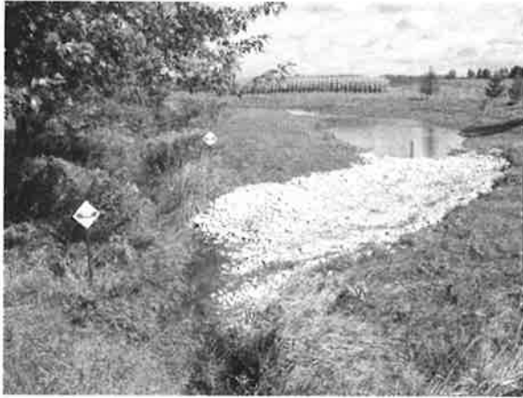
Figure B7-2. An off-line sediment trap.
