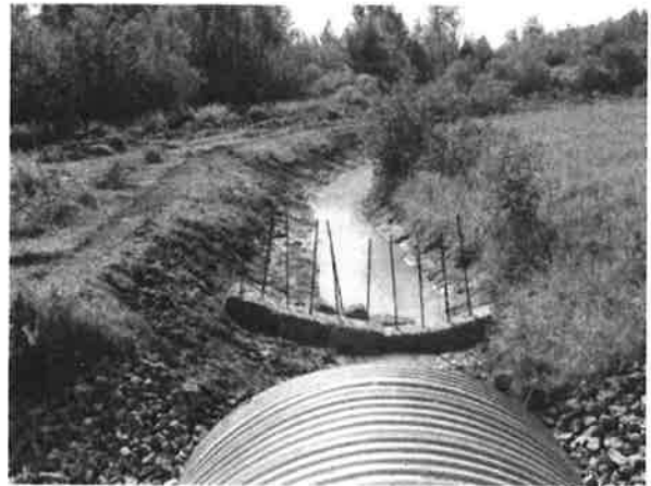
Figure B6–2. A straw bale check dam.
