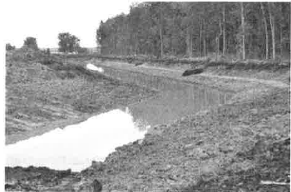
Figure B11–12. A dewatered channel with root wads on a littoral shelf.
