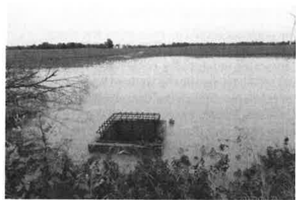
Figure B8-4. A water retention area.
