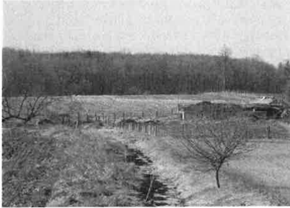
Figure C3–2. A drain set back from a nutrient management storage facility.
