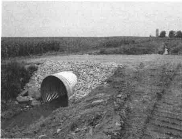
Figure B1–1. Rural drainage works.
