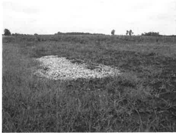
Figure B10–21. A blind inlet in a field.
