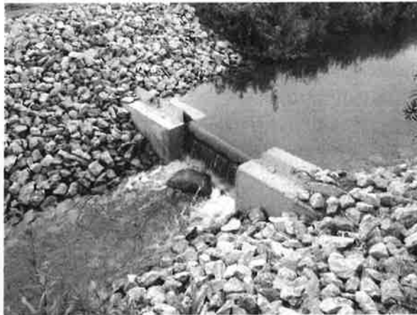
Figure B10-27. A small dam.
