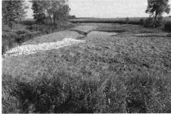
Figure B7-3. Straw/hay mulch spread on exposed soil surrounding a sediment trap.
