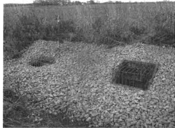
Figure B10–19. Birdcage grate with stone apron.
