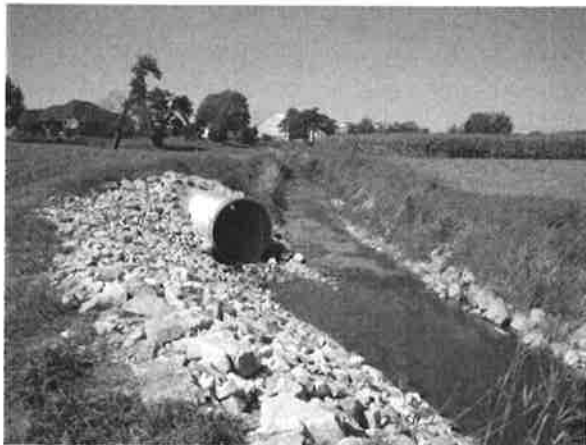
Figure B2–2. Example of a good outlet.
