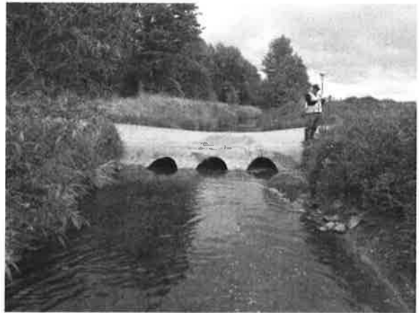
Figure B10-8. A low-flow crossing.
