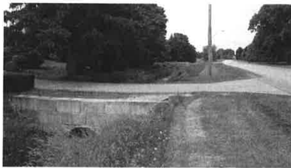
Figure A9-5. A private crossing with an asphalt surface (side view).
