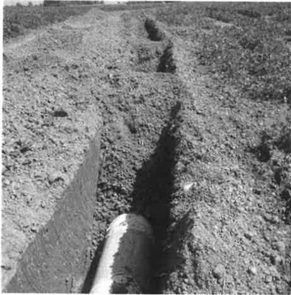
Figure B10-13. Installed concrete pipe (with geotextile-wrapped joints).
