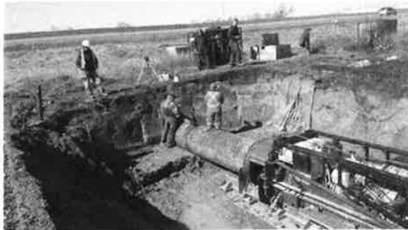
Figure B10–5. A trenchless crossing.
