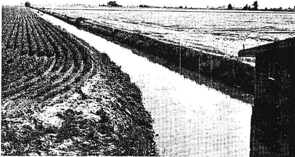
Inlet channel and pumping installation.
