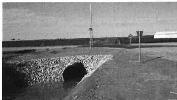
Figure B10–2. An embedded culvert.
