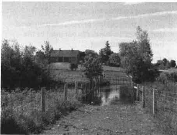
Figure B10-7. At-grade or bed-level crossing for livestock.
