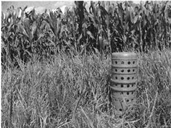
Figure B10–16. A riser inlet installed at the edge of a field of corn.
