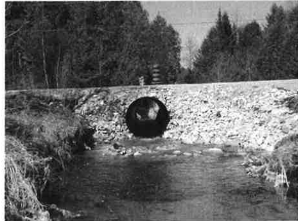
Figure C9–4. A large-diameter culvert on a non-listed waterway.
