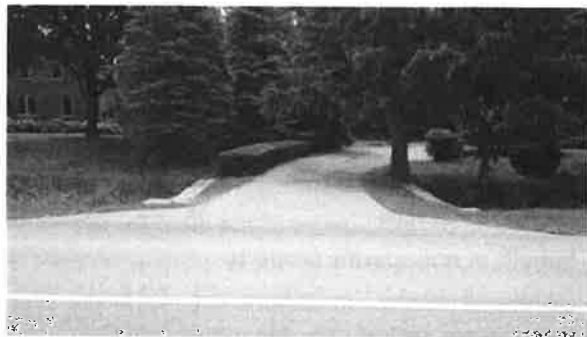
Figure A9-6. A private crossing with an asphalt surface.
