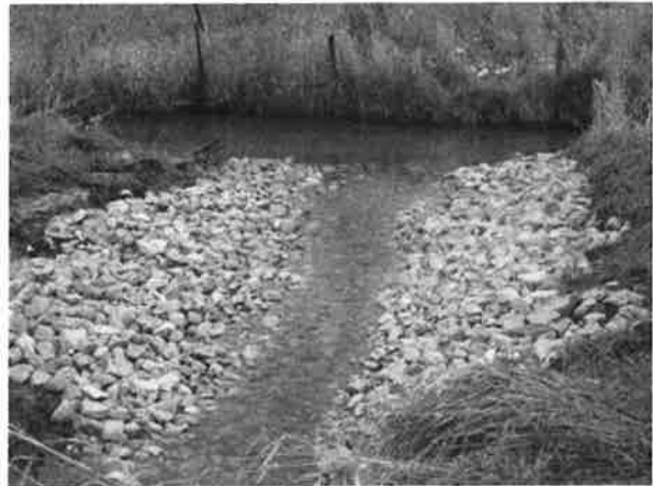
Figure B7-5. Riprap armouring of a drain.
