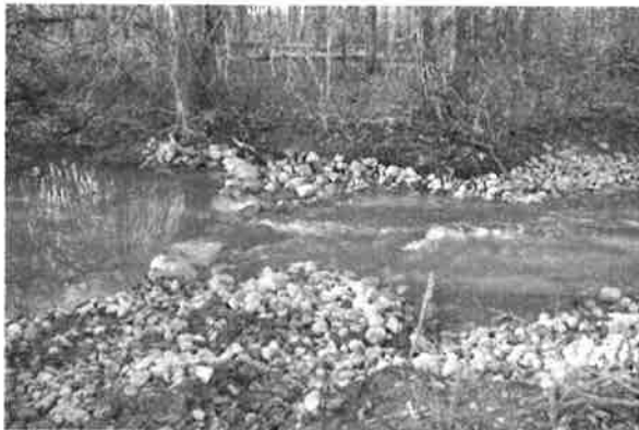
Figure B3–6. A Newbury weir.
