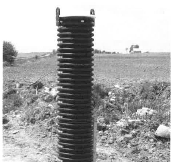
Figure B11-17. A controlled drainage structure prior to installation.
