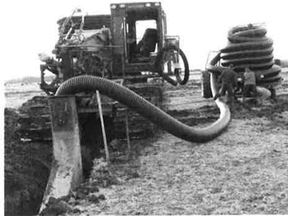
Figure B3–1. A contractor installing a rural piped drain.
