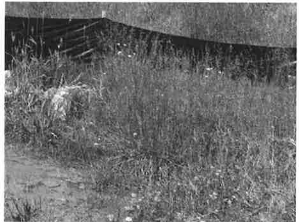
Figure B6–3. A silt fence installed next to a drain.
