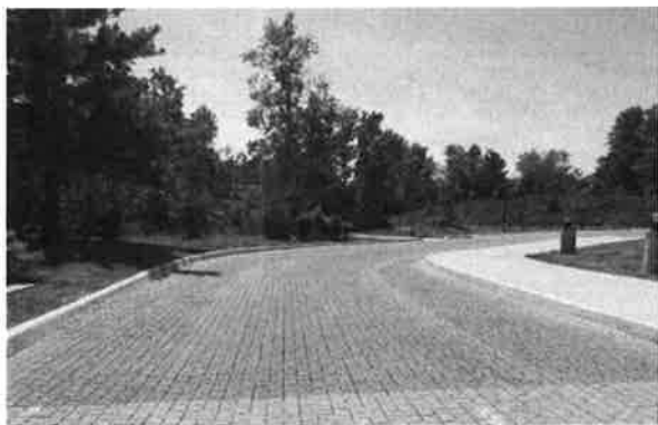
Figure B5-2. Permeable paving is used to increase infiltration of water.
