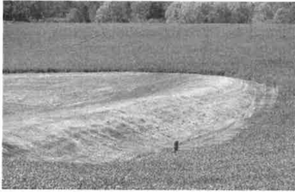
Figure B11-15. A WASCoB with berm and inlet.
