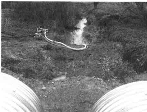
Figure C3–1. Dewatering for a culvert installation.
