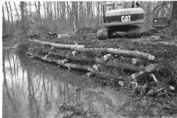
Figure B11-8. Construction of a live crib wall.
