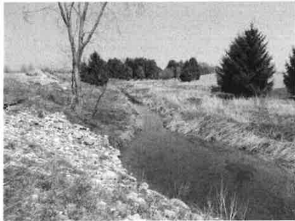
Figure B7–1. Riprap placed at the bend of a drain.
