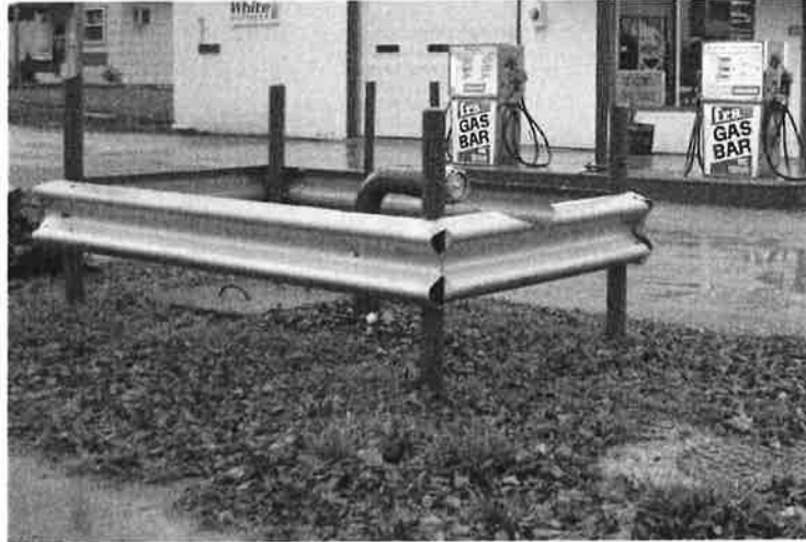
Highgate Cistern Storage Tank
