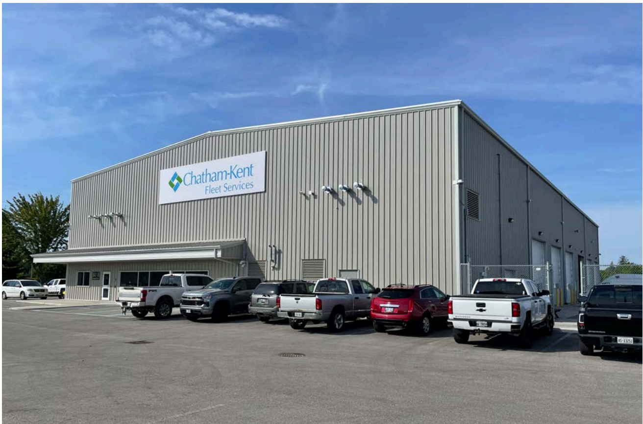
Chatham-Kent Fleet Garage
