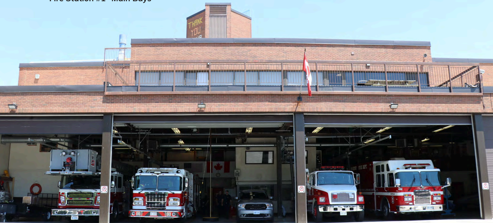
Fire Station #1- Main Bays
