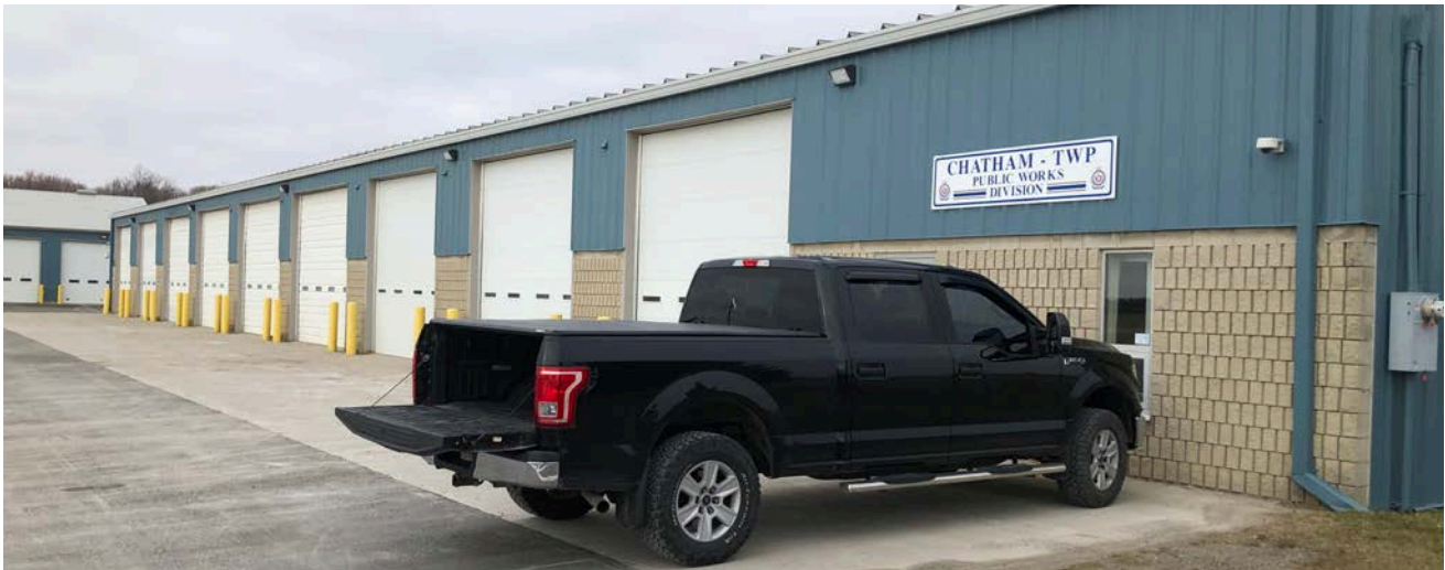
Chatham Township Public Works Garage
