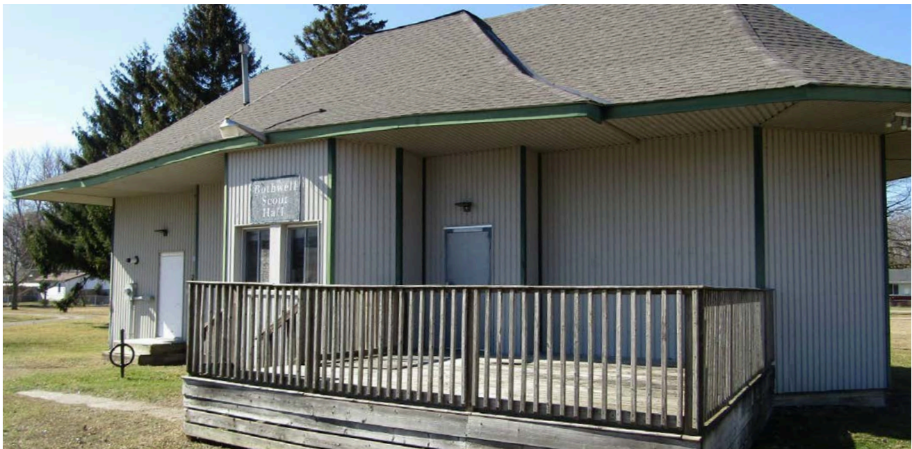
Bothwell Scout Hut, Bothwell
