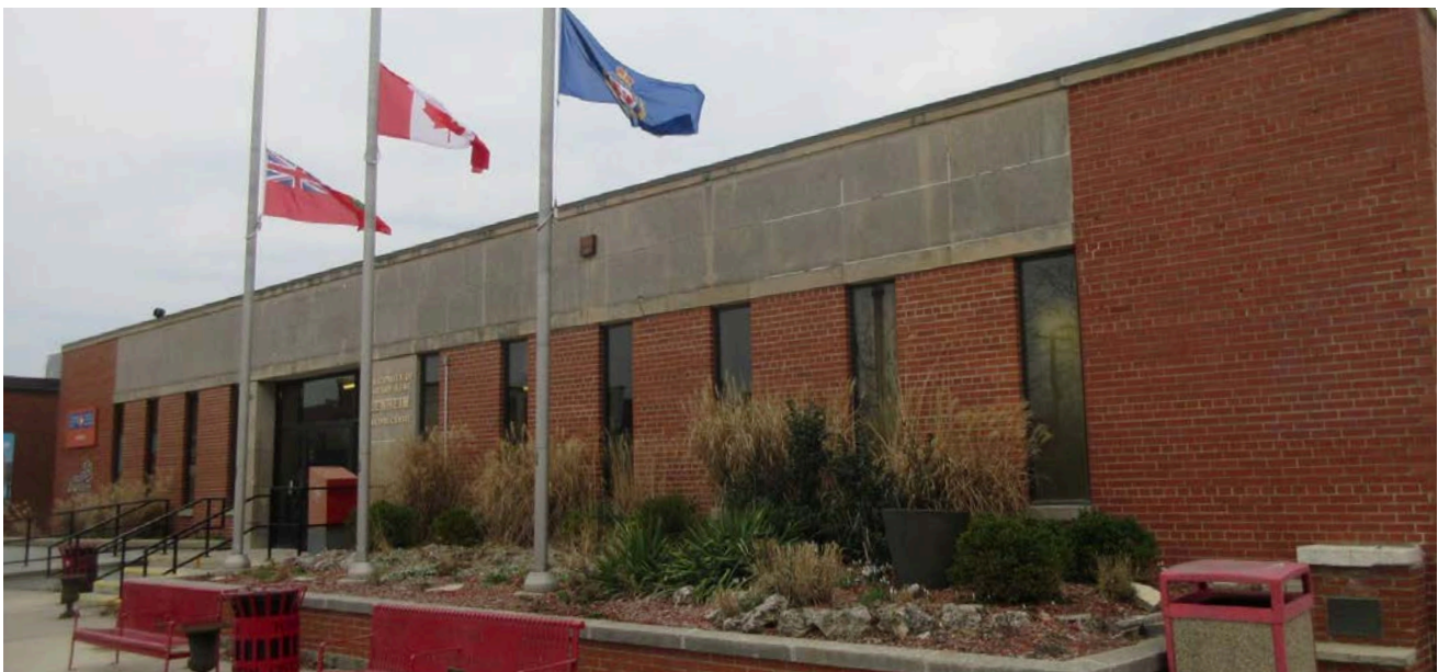
Blenheim Service Centre
